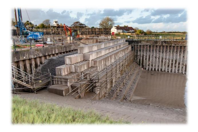
Following completion of the relieving slab, we'll be removing the legato wall (pictured above) which was in place to support the removal of the old abnormal loads quay.
