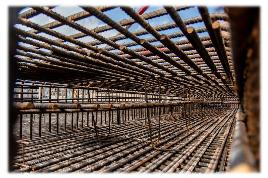
Concrete will be poured into this large structure, which will form the relieving slab – the area where large components will be offloaded from vessels
